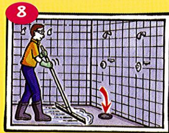
8 Squeegee excess moisture to floor drains.
